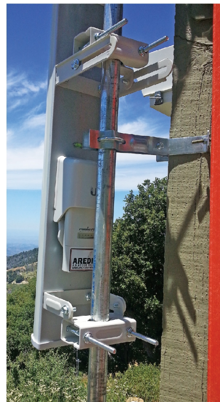
Figure 2 — A 3.4 GHz downlink from a backbone node uses a 120° sector antenna. [Andre Hansen, K6AH, photo]
